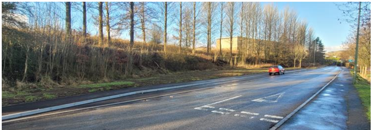
Fig 20 showing recently constructed drop-off zone/bays to the rear of the site at Allotment Road.
